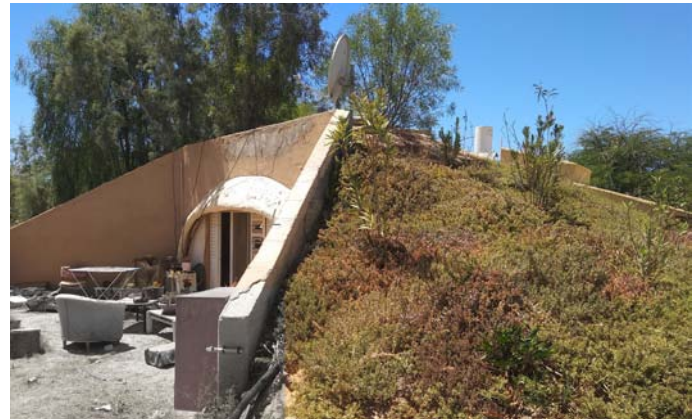
In the early 1980s Givoni’s experiments at the Institute for Desert Research included an earth-sheltered dome, which continues to house residents and harbor vegetation.
