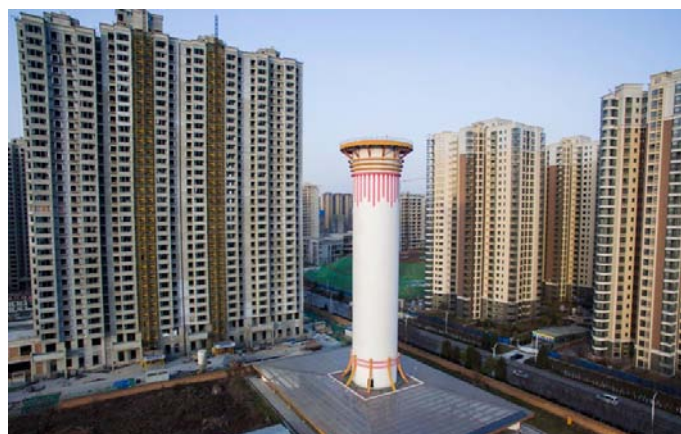
A 100-meter-tall air purifier in Xi'an City, Shaanxi province, Jan. 17, 2018. Source: www.sixthtone.com
