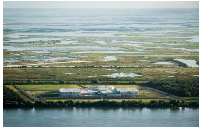
The Plaquemines Parish Detention Center was rebuilt for $105 million in a Louisiana marsh that had been ravaged by Hurricane Katrina. Source: nytimes.com
