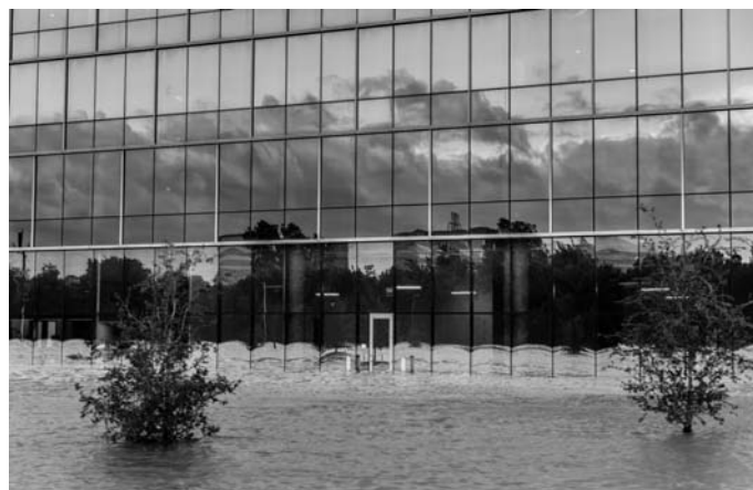
A flooded office building in the Energy Corridor. Source: https://www.bloomberg.com
