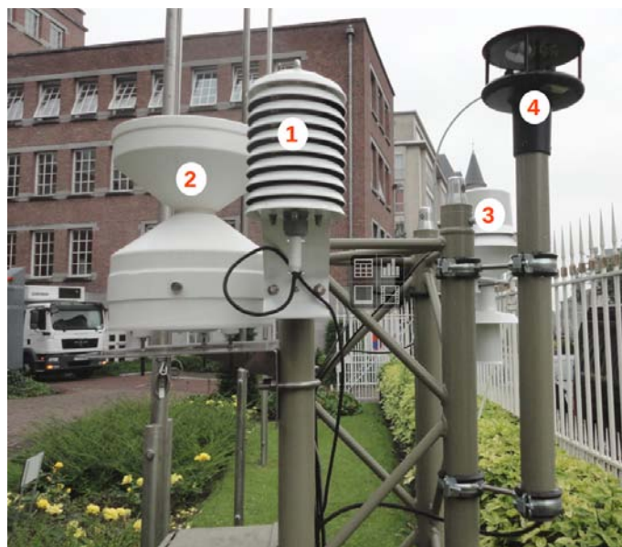
Figure 4. Detailed view of the sensors at one of the weather stations: passively ventilated radiation shield (1) with temperature and relative humidity measurement, rain gauge (2), actively ventilated shield (3) with temperature sensor, and sonic anemometer (4).
