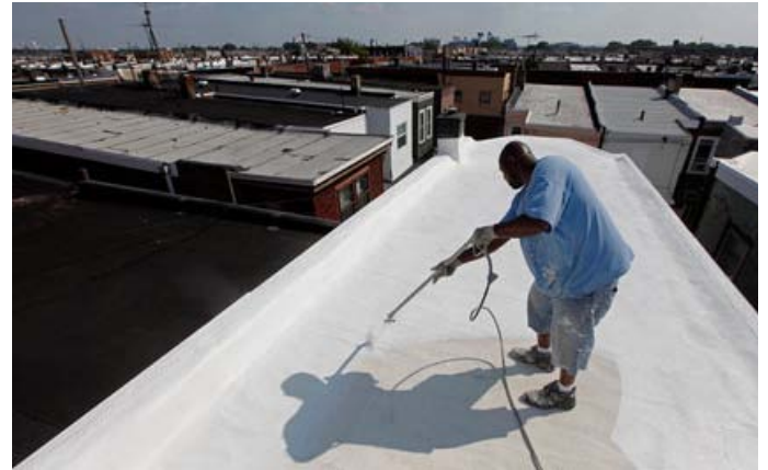
Painting a roof white in Philadelphia. ( NYTimes )
