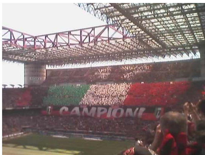
Figure 1. The San Siro Stadium in Milan. Note how the roof structure and tall stands combine to reduce direct sunlight reaching the pitch. In the 1980s and '90s, the resulting poor turf quality was a serious issue of concern (Source: Wikimedia).
