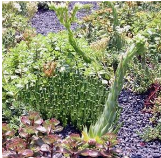
Plants growing on the roof of the Montgomery Park Business Center, Baltimore, Maryland (Photo courtesy of the National Renewable Energy Lab)
