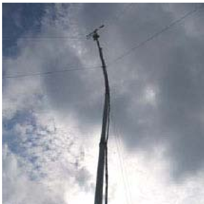
Figure 5. Pneumatic mast with eddy covariance sensors at top and permanently bent middle section.
