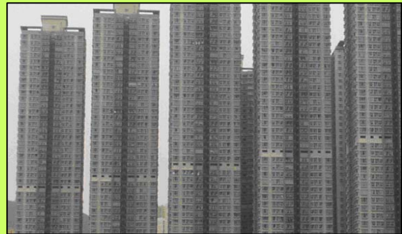
Figure 3: Tall buildings too closely pack together creating an 'effective' wind block to the city behind.
