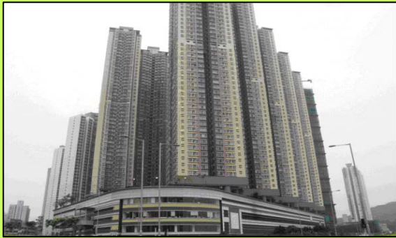
Figure 2: A typical building morphology in Hong Kong: tower blocks sitting on a podium that occupies the entire site. When podiums are very close together, they significantly reduce the air space at pedestrian levels.
