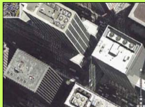
Fig 3. Individual dwelling air conditioning units in Hong Kong (above) and rooftop building units in New York (from Google Earth). There are in NYC alone, 6000 high rise, and 10 000 medium rise (approx 10 stories) buildings that are all pumping out such concentrated heat, not to mention all the individual window air conditioners.
